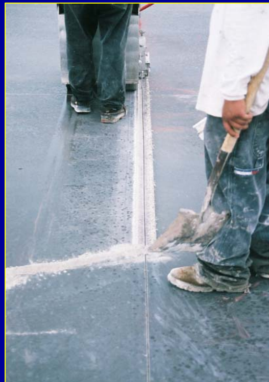
THE FINISHED JOINT
