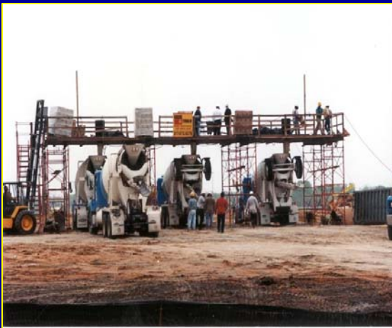
LOADING FIBERS ON PLATFORM
