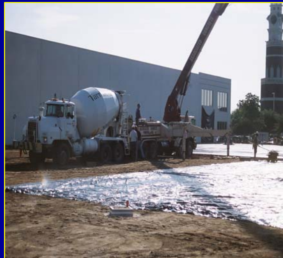
CONCRETE BEING PUMPED
