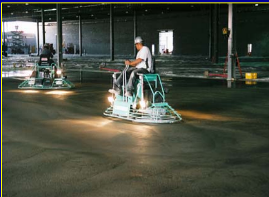
SFRC BEING FINISHED WITH PANS
