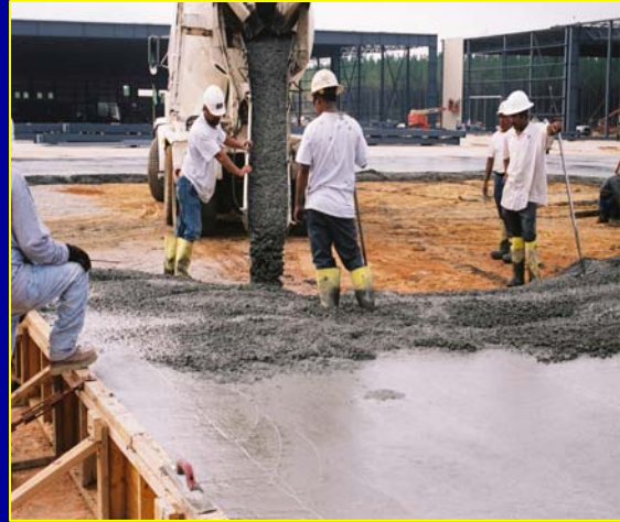
CONCRETE BEING TRUCK DUMPED
