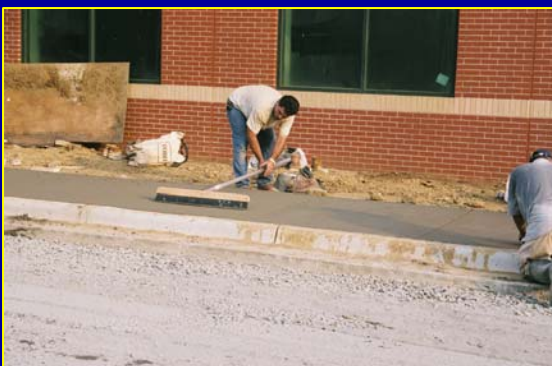
BROOM FINISH AND TOOLING JOINTS
