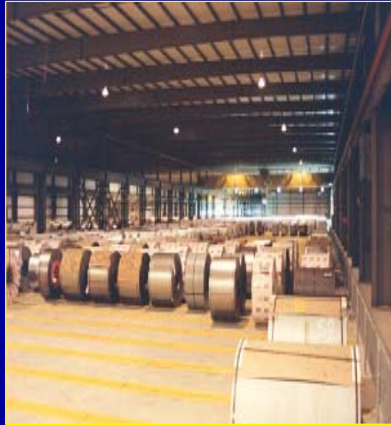
FINISHED STEEL PROCESSING PLANT
