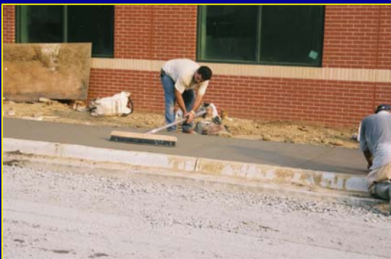
BROOM FINISH AND TOOLING JOINTS
